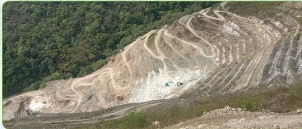
SMCL starts operation of Kothagpa Gypsum mine, Pema Gatshel
