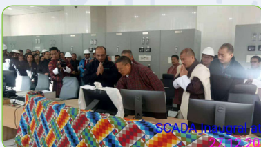
SCADA commissioned at KHP by DGPC
